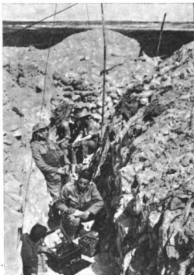
A Trench Station.
